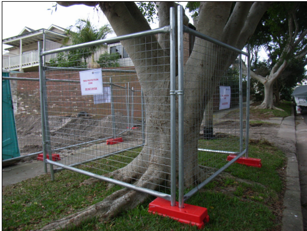
FIGURE 1.5 Tree Protection Fence on Nature Strip
